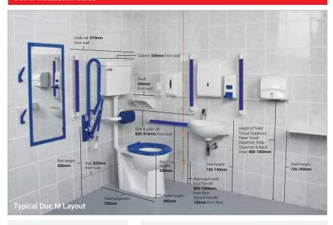
It is essential that wheelchair users are able to approach, transfer to, and use the sanitary facilities provided within a building. This means a wheelchair-accessible unisex toilet must be made available.
