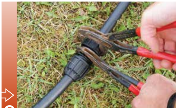
7 Tighten with a wrench.
