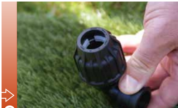
5 Screw on the nut just until it stops, do not tighten fully at this point
