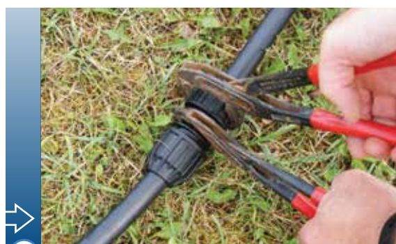
8 Tighten with a wrench
